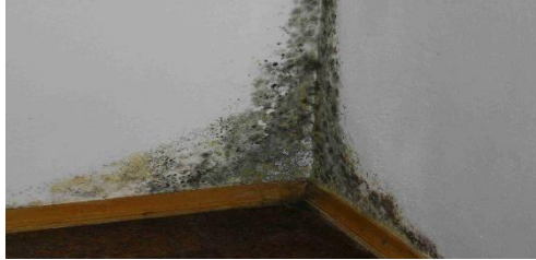
Figure 5 – Biological corrosion in animal farm
