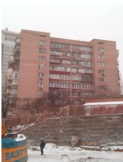
Fig. 1 – Investigated building and retaining wall view
