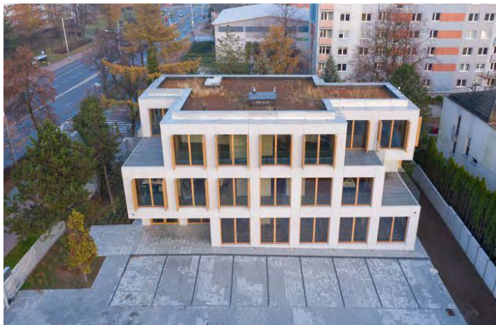
Fig. 9. Green roof over the EXG office building in Czestochowa [23]
