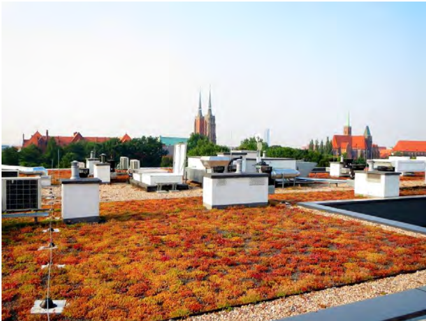
Fig. 4. Green roof at Botanica Residence in Wroclaw [18]
