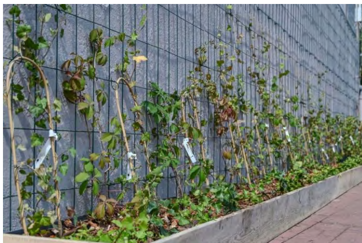
Fig. 10. Green facade created on the external wall of the City Hall building in Czestochowa [24]
