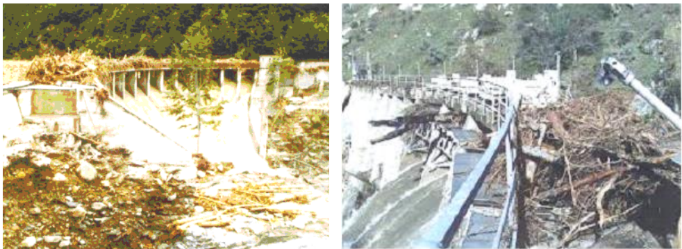
Fig. 2 – Overtopping of Palagnedra dam in Switzerland due to plugging of spillway by floating debris in 1978 (left) [27]; the similar plugging of the spillway of Kerckhoff dam in California, USA, in 1997 (right) [28]
