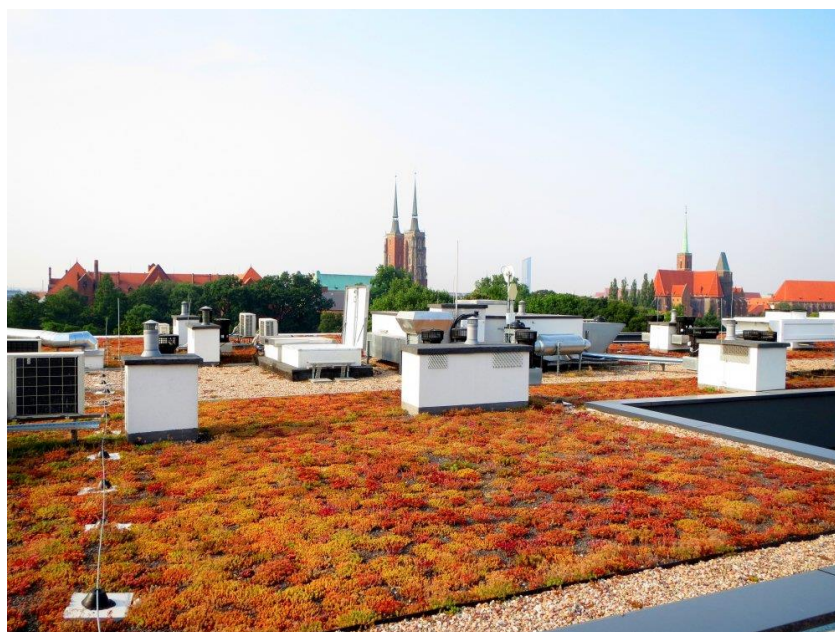
Fig. 4. Green roof at Botanica Residence in Wroclaw [18]
