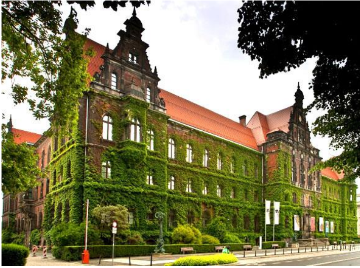
Fig. 5. Green facade on the building of the National Museum in Wrocław [19]
