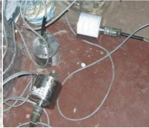
Fig. 6 – Vibration sensors № 4 and № 5 for registration of oscillations of the top 9 th floor of the building towards X, Z or Y, Z directions
