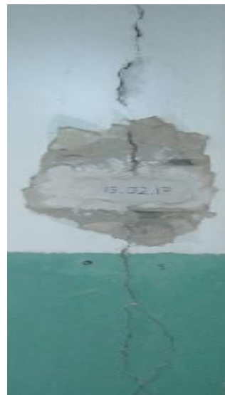
Fig. 2 – Chalky screed state after pile installation
