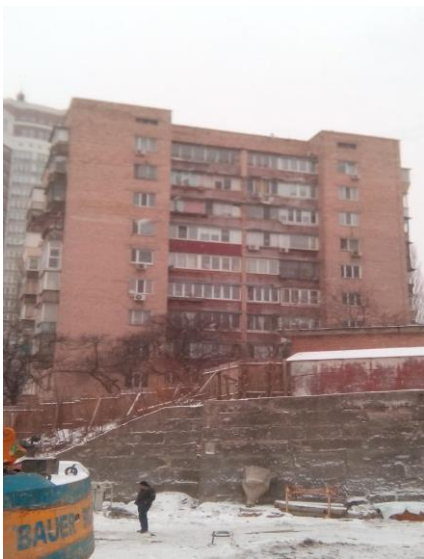
Fig. 1 – Investigated building and retaining wall view
