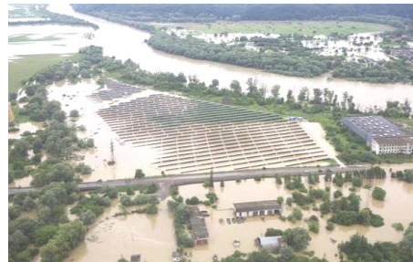
A flooded solar power plant
